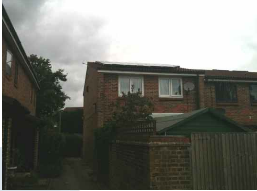
The light sensor mounted on the side of one of the houses
