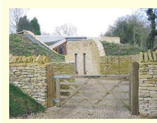
After excavating the plot and drilling two boreholes for heat extraction, a reinforced concrete foundation raft was laid, supporting the walls and flat roof, also of reinforced concrete. The structure was waterproofed and the earth replaced above and around the house on three sides. This was topped with a multi layer insulating and waterproofing umbrella spreading out 3 metres beyond the house to trap heat within the
