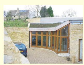
The behaviour of the four rooflights was unexpected as they appear to behave just like any conservatory, losing heat rapidly as temperatures drop, and rising just as rapidly when the sun comes out. Our temporary solution this 2004-5 winter has been to fit insulated wooden shutters in each well.
